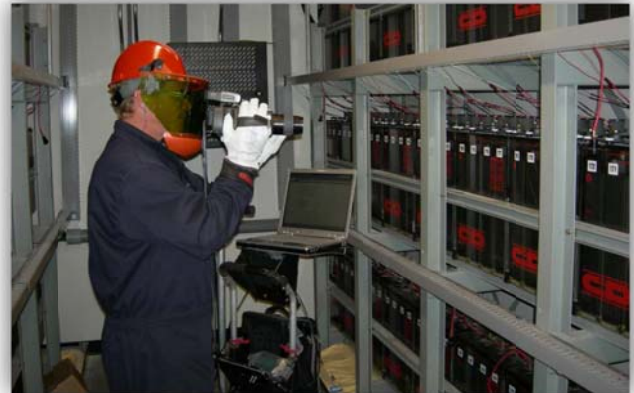
Figures 8a & 8b) Safety around electrical equipment is the #1 consideration during infrared surveying. Some of the options: 8a shows an IRISS infrared window installed in electrical cabinet 5 . The thermographer safely holds an infrared camera up against a viewing port or window to see inside the switchgear. These windows can be custom fit to any data center equipment. 8b) Thermographer wearing proper personal protective equipment (PPE) inspecting a battery bank during a full battery discharge test.
