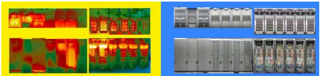
Figure 6a) Zoomable thermal map imagery server racks (overview).
